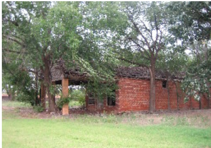
Old abandoned country store in Beckham County, OK
